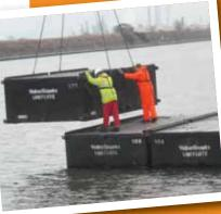
Structural Soils is mooring two barges and platforms in the estuary from which it will drill a series of up to 22 boreholes up to 45m beneath the riverbed of the proposed second crossing from Runcorn to Widnes.
